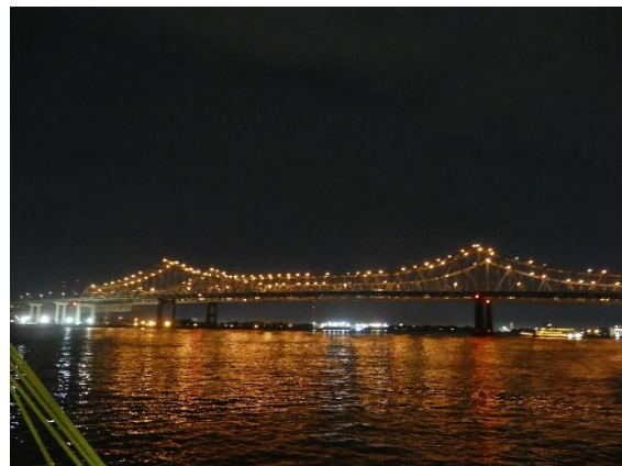
The Bridge over the River (looking upstream)
