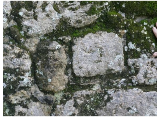
Up close view of the mortar
